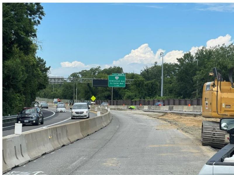
HREL 4C median crossover construction
